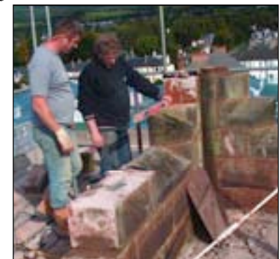
Working at the top of the tower
