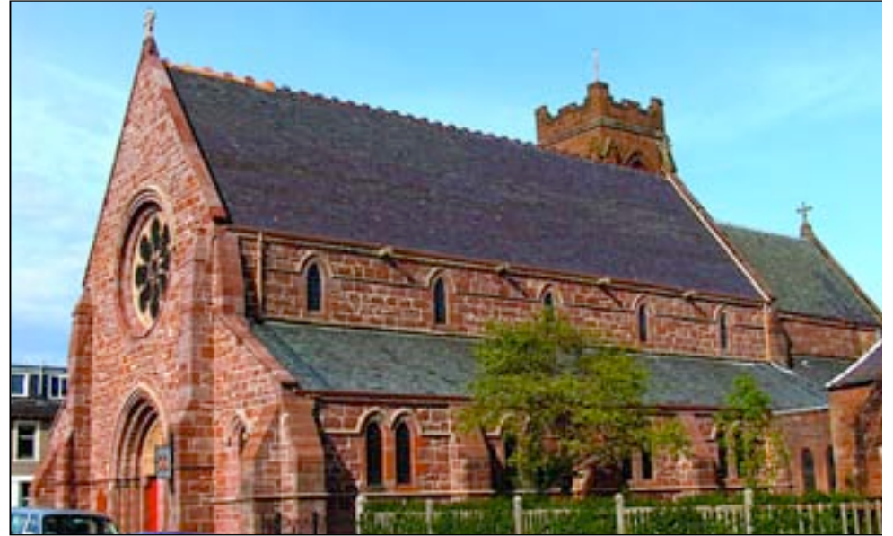
The church from the south west after the first phase of restoration
