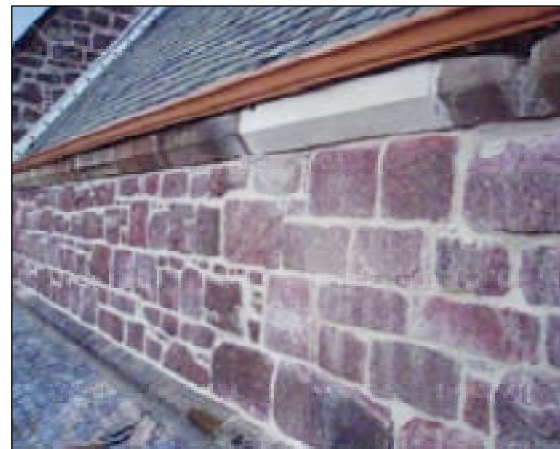
The restored wall - left
