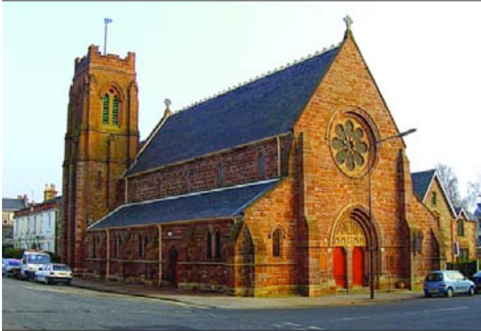
The church from the north- west after the second phase of restoration, May 2006
