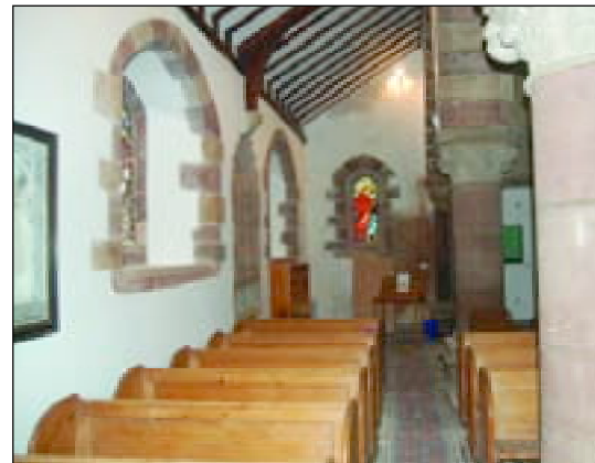
Left - South Aisle nearly finished
